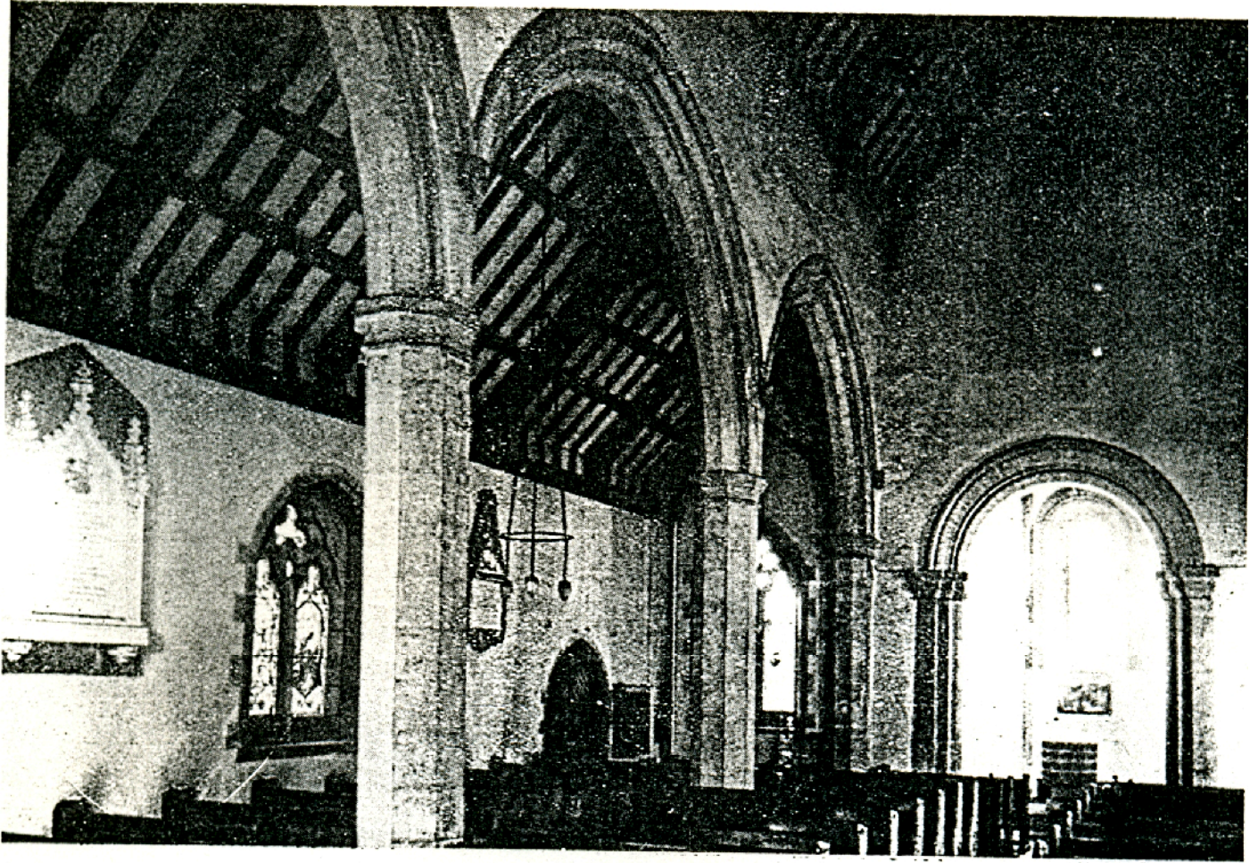
BRAMHAM CHURCH: SOUTH ARCADE AND (MODERN) TOWER-ARCH AND FONT.
